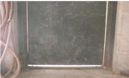
Figure 8: Air leakage can occur because gaps lead to uncontrolled migration of conditioned air through the building envelop (Goal #2).
