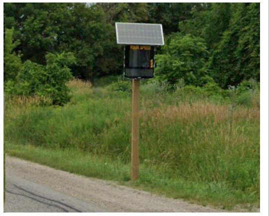
TYP. Radar Speed Sign Placement
